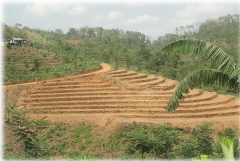
Photo: Zauthangvunga Terrace at Darnam Zau- After Completion
